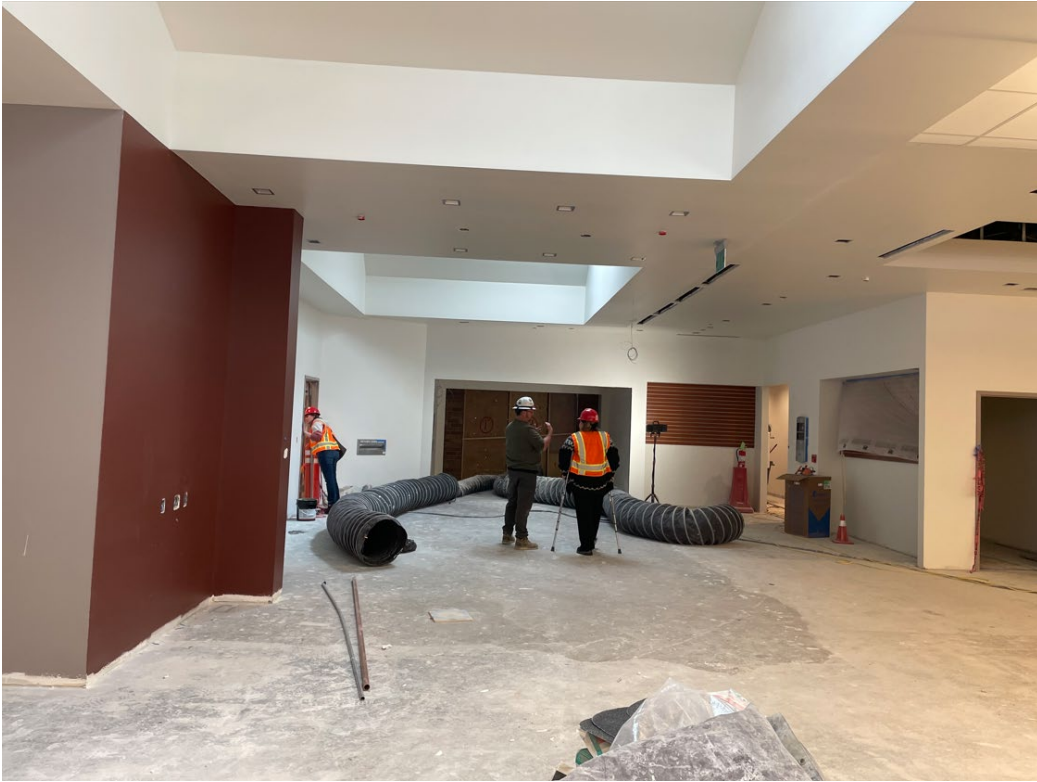
Front Entrance ready for doors & carpet.
