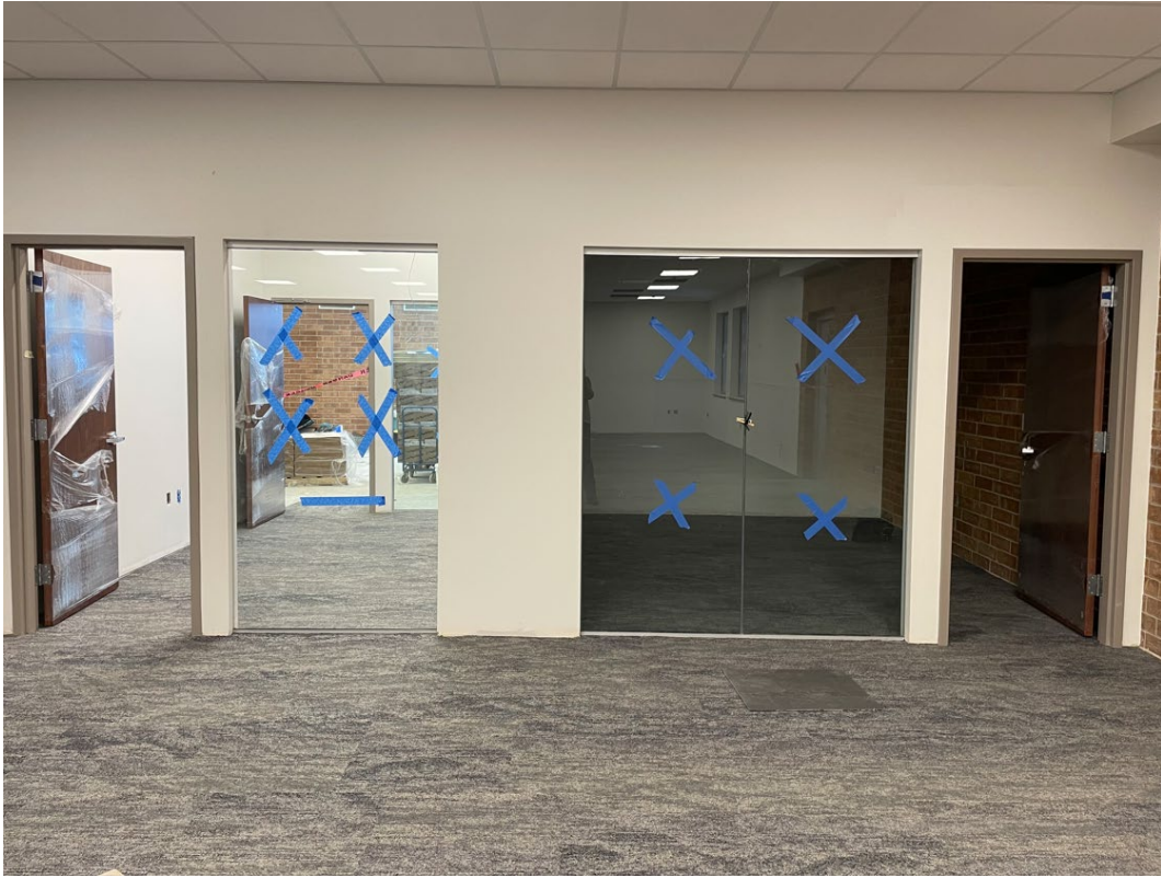
Offices almost ready!
