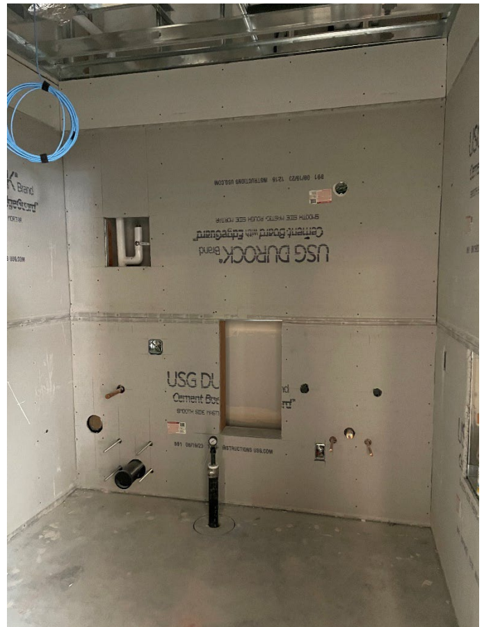
Toilets ready for Tiling
