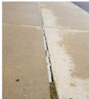
C. Pavement Settlement
