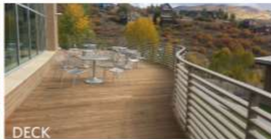
Addresses site issues: F & E
