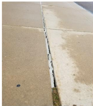
C. Pavement Settlement
