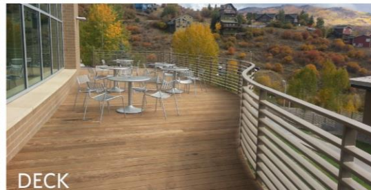
Addresses site issues: F & E
