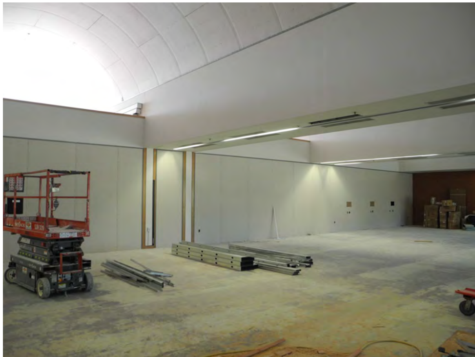
Installation of interior drywall in early July
