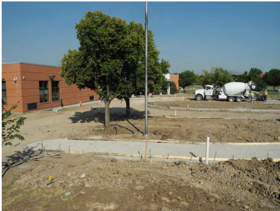
Overall view of new drop-off loop. Note installed curb/gutter.
