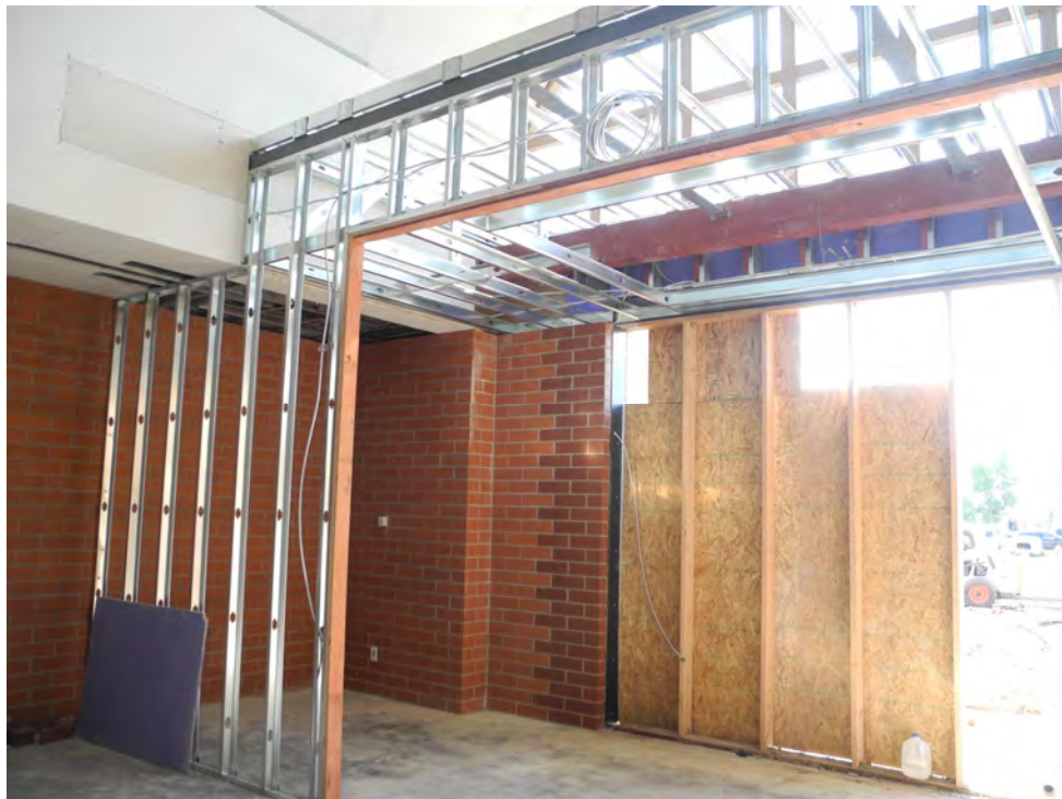
Framing at new entry vestibule
