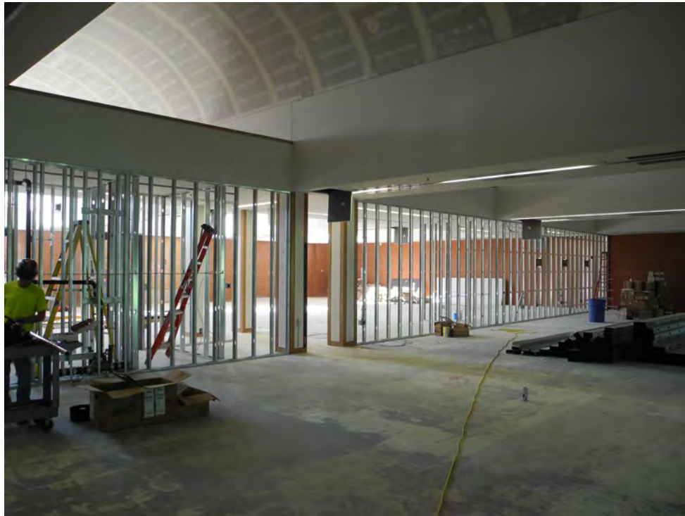
Beginning of interior framing in mid-June
