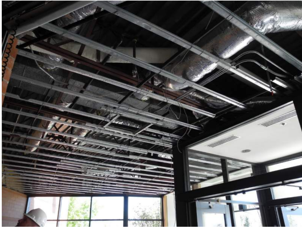
Ceiling at old entry location has been removed, exposing HVAC ductwork
