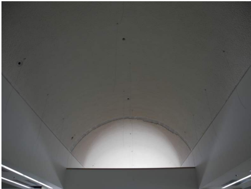
Previously installed hanging light fixtures have been removed, exposing the full barrel vault ceiling
