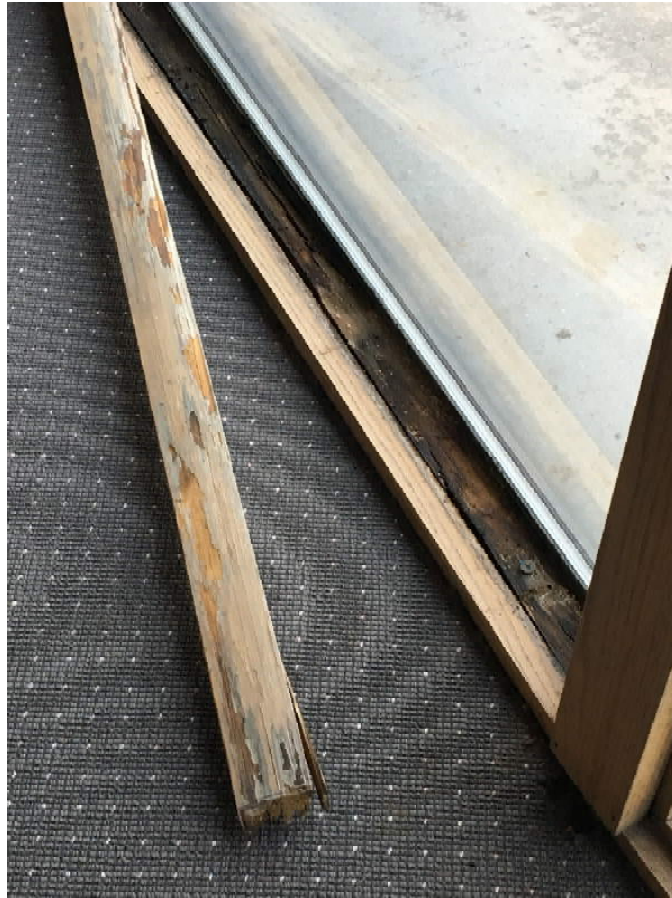
Damage at wood window sill
